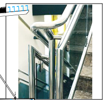
5. STAIR BALUSTRADE Stainless steel
